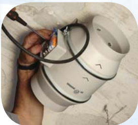
Carry out the wiring connections
