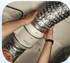
Connect the ducts
