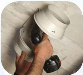
Fix the support bracket
