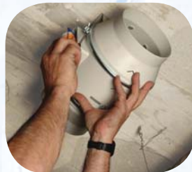
Place the impeller and motor assembly
